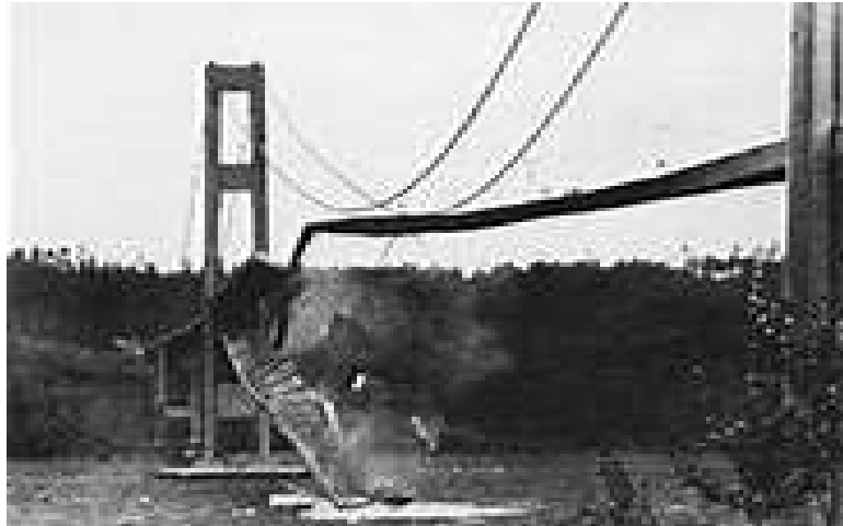
Figure 3: The collapsed Tacoma Bridge
