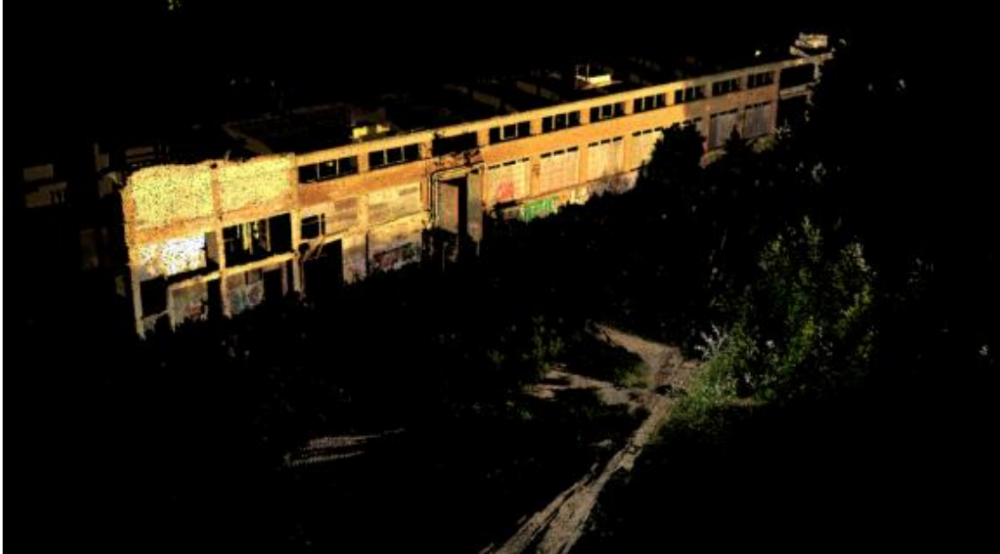
Figure 12. Outdoor scan point cloud.
