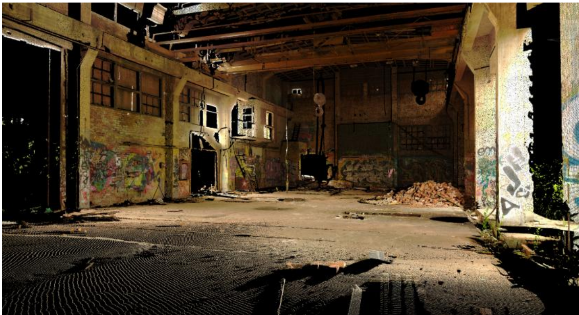
Figure 11. Indoor scan with Outdoor HDR setting from other point of view.
