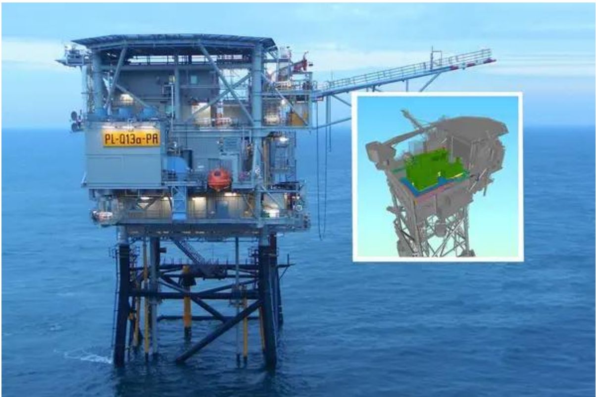
Figure 5. Neptune Energy's Q13a-A platform (Nel Hydrogen, n.d.)
