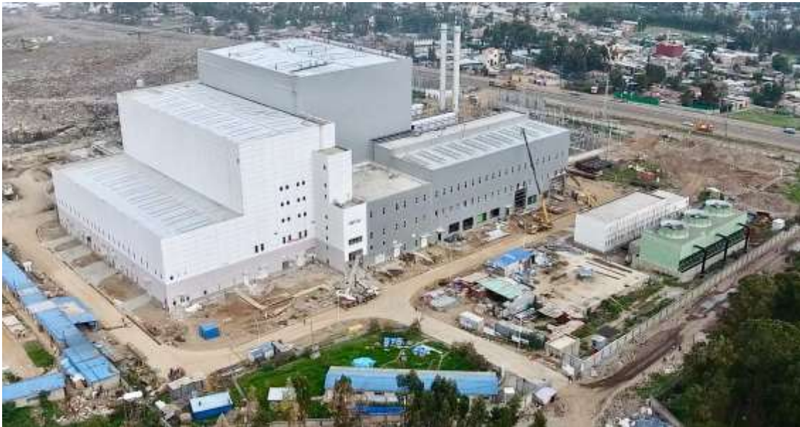
“Fig. 10.” Construction of the Reppie Incineration Plant in Ethiopia.
