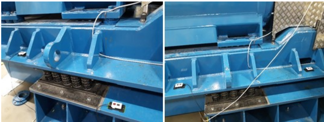
Figure 4. The Bosch XDK110's at their original orientation and position (left) and at their final installation (right).
