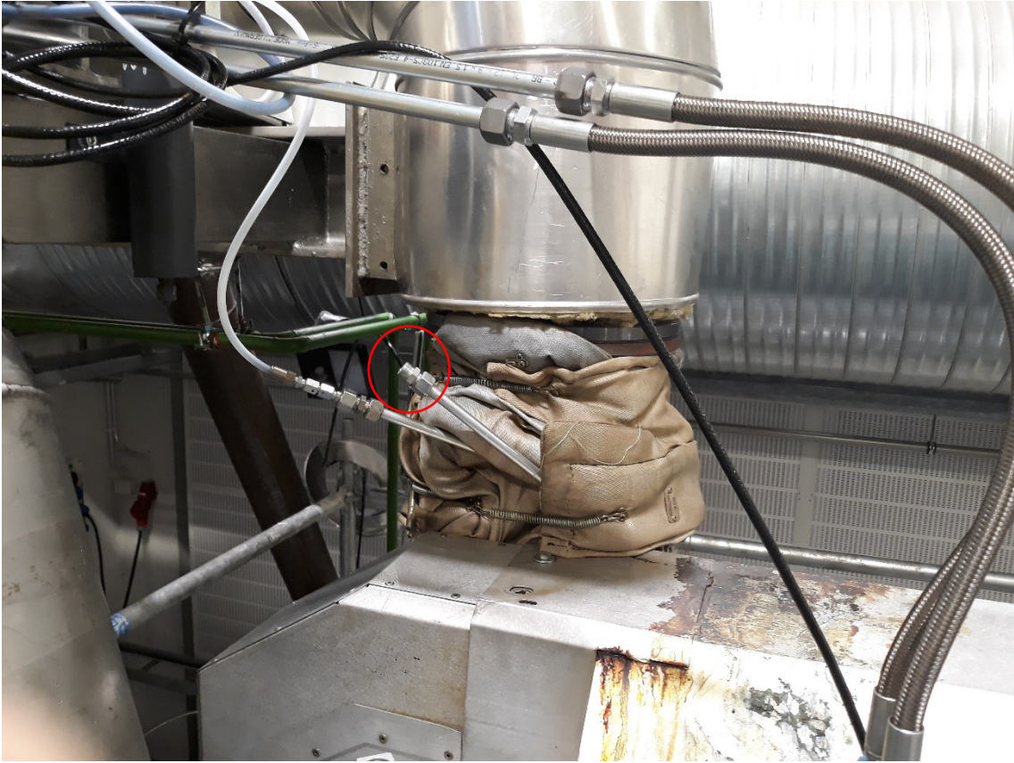
Figure 8. A closeup of the exposed connector to the engine's internal exhaust gas system, circled in red.
