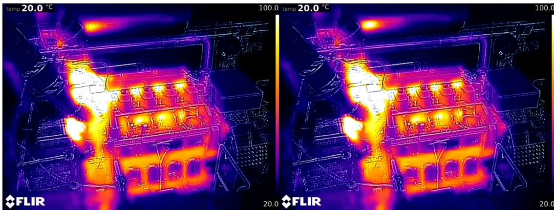
Figure 15. Temperatures 10 minutes after the load command to 100 % in the second experiment. No leakage on the left, artificial leakage on the right.
