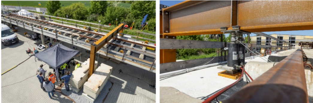
Figure 7: IDA-KI OpenLab Bridge During Load Test Phase.
