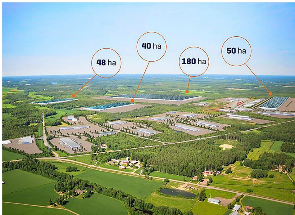
Fig. 2. A future industrial site for the construction of battery plants (Photo: modified and reproduced with permission from a downloadable brochure titled ‘Establishing a battery factory’, produced by GigaVaasa in 2019 (GigaVaasa 2022))
