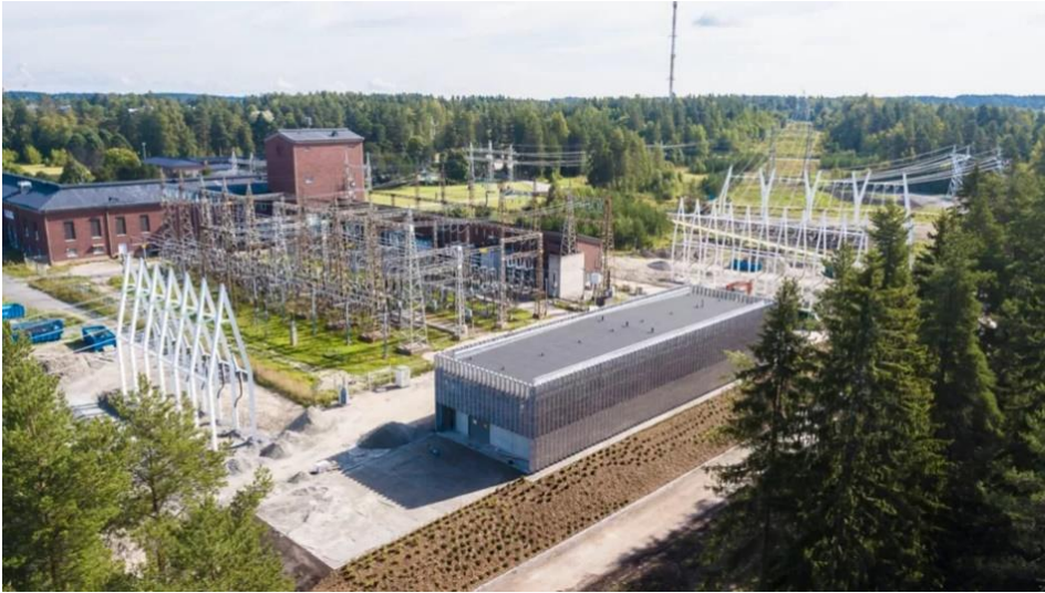
Figure 1 Substation in Finland (Hitachi Energy, 2020)
