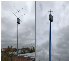
Figure 35. Winkler Turnstile VHF and UHF Antennas at the University of Vaasa Premises.
