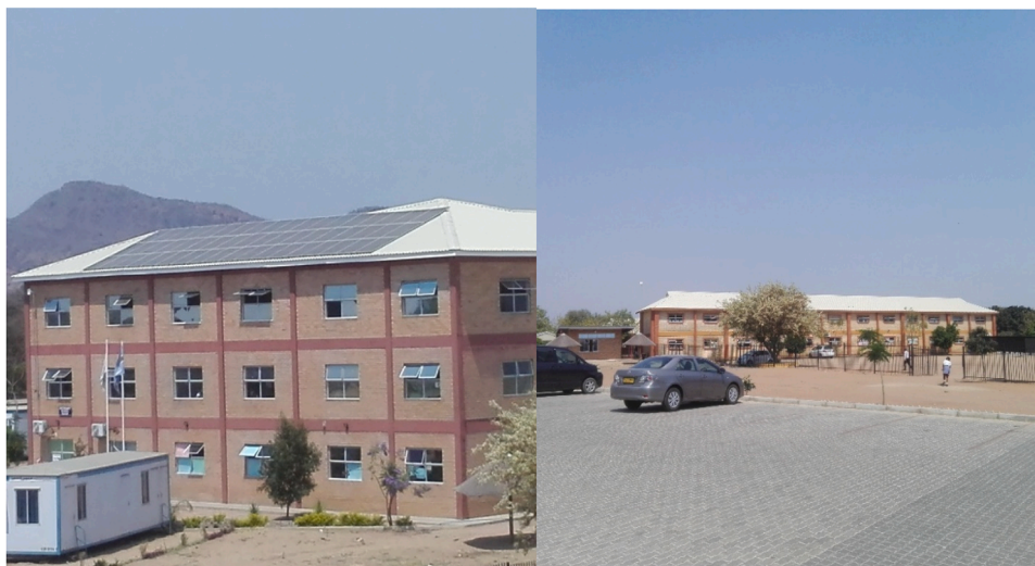
Fig. 4. Regent Hill School energy village.
