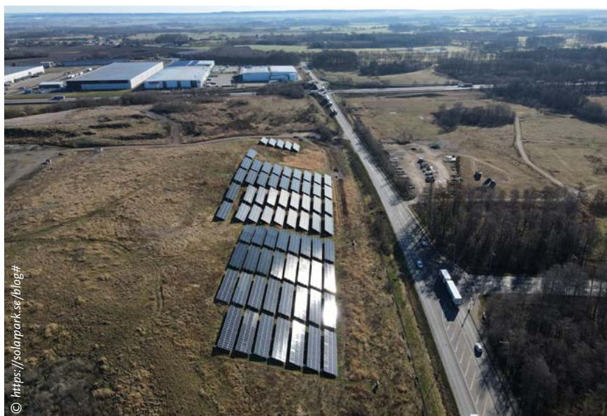
FIGURE 4: PV park Solar Park in Helsingborg, Sweden.
