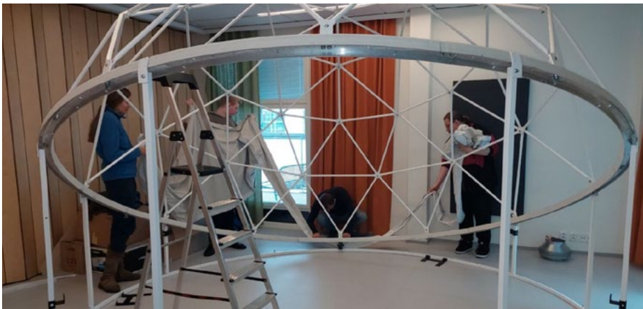
Picture 38. The completed dome structure looks like this (photo: Martta Niemi).
