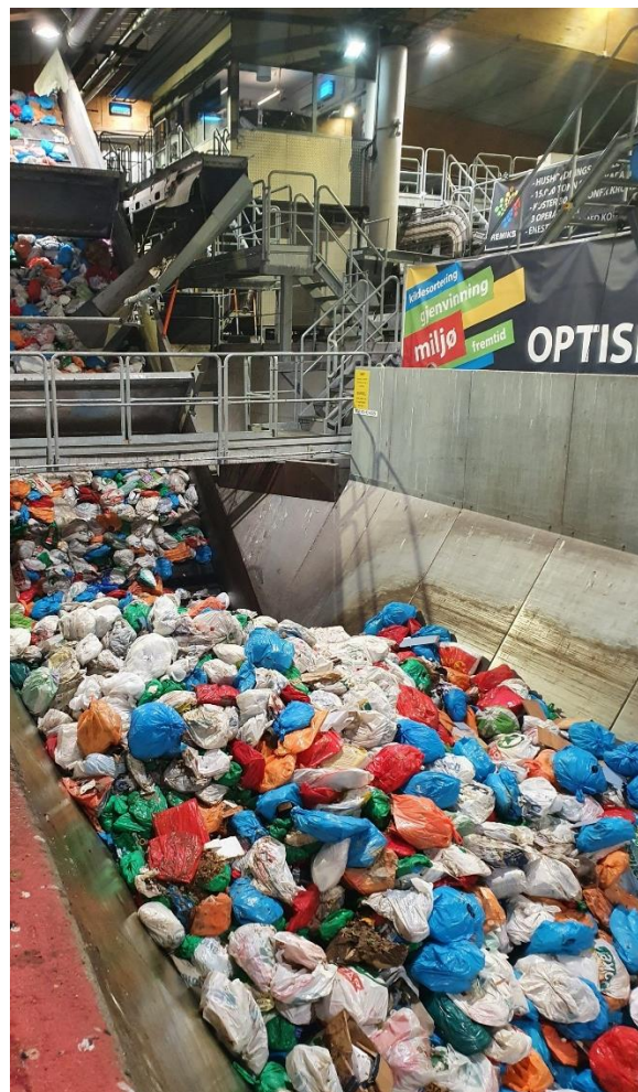
Figure 5: The Remiks optical waste sorting facility in Tromsø
