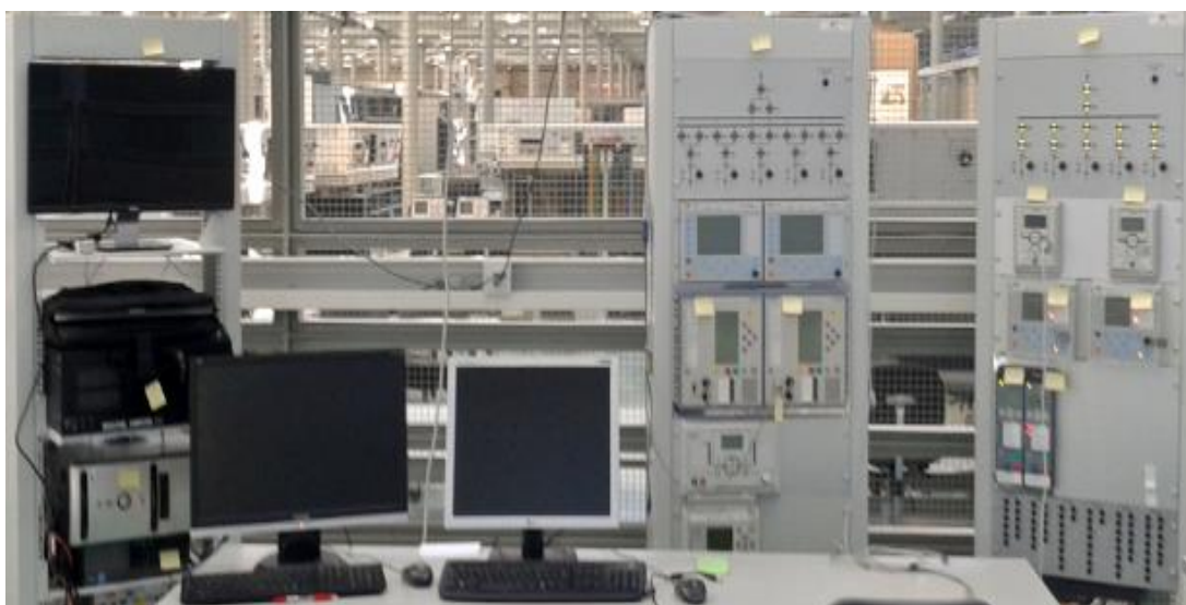
Figure 22. The DEMVE project, a section of the Technobothnia laboratory.
