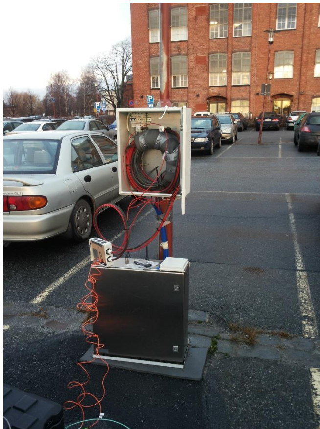
Picture 1. Parking lot with vertical optical fiber cables underneath.
