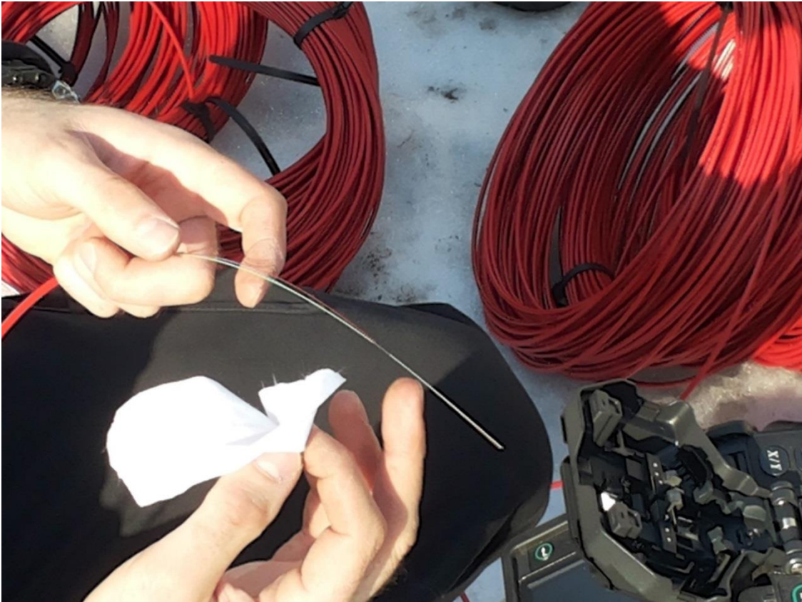
Picture 6. The making of fusion splice. Bottom right is the splicing device.
