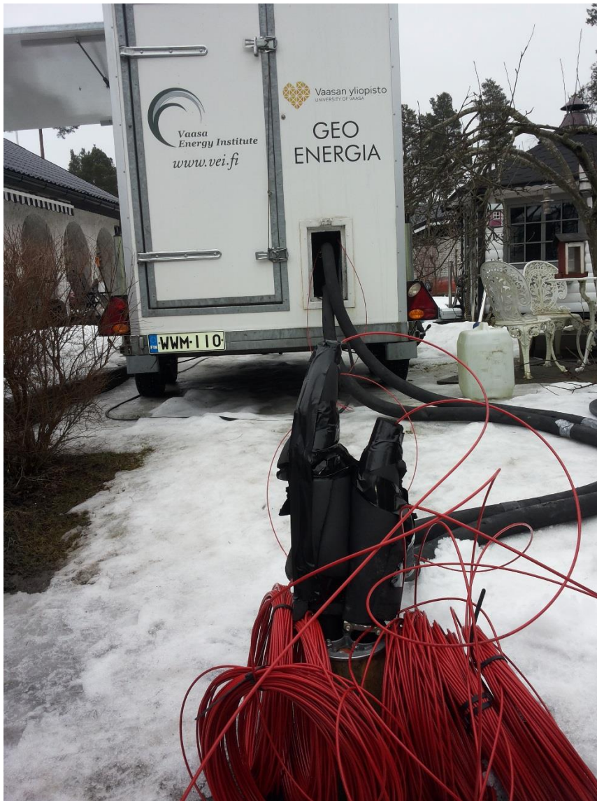
Picture 8. Pipe insulation featuring optical fibers.
