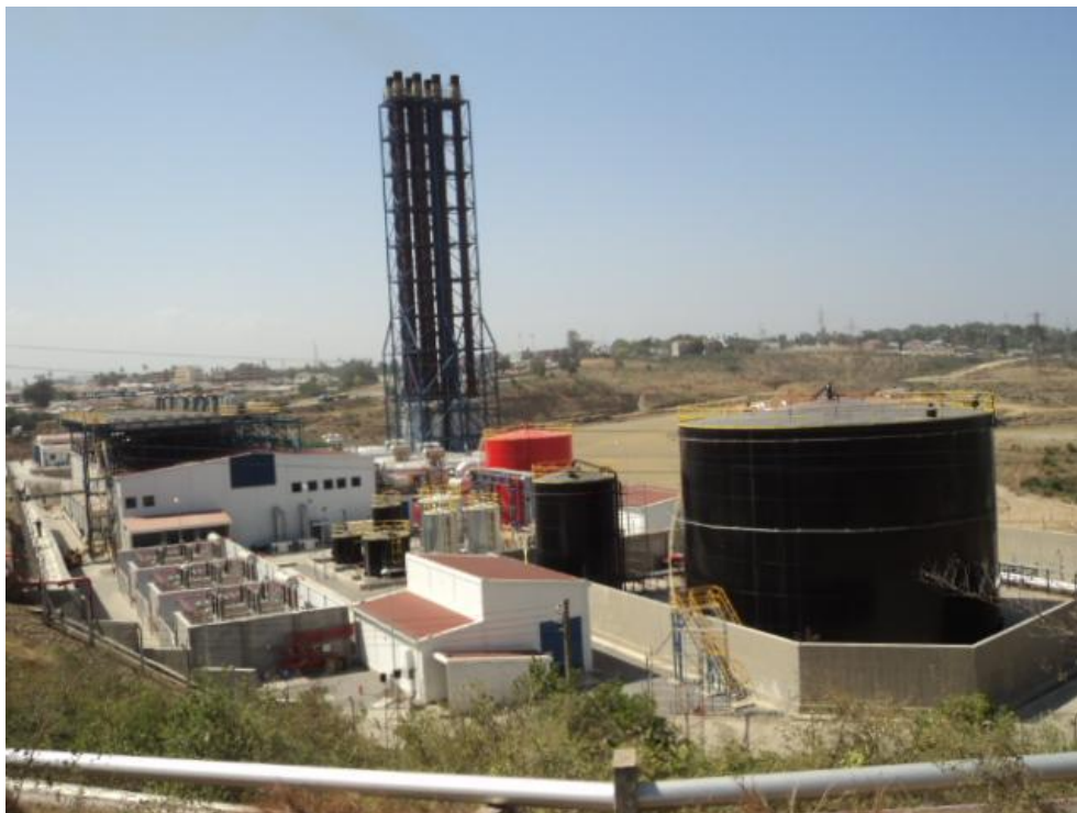
Figure 1. Kipevu III power plant constructed by Wärtsilä Oy to KenGen (KenGen 2013).
