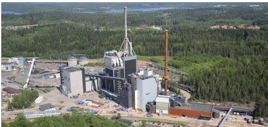
Figure 2. Kymijärvi power station area in Lahti, Finland. The highest construction is disused coal power plant Kymijärvi 1. On the left side of Kymijärvi 1 is gasification power plant Kymijärvi 2 which has generated electricity and district heating since 2012. In the foreground of the picture is biopower plant Kymijärvi 3 which has produced district heating since 2019. (Lahti Energia, 2020)
