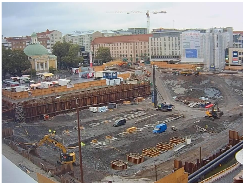
Fig. 6. Toriparkki construction site at June 2019.
