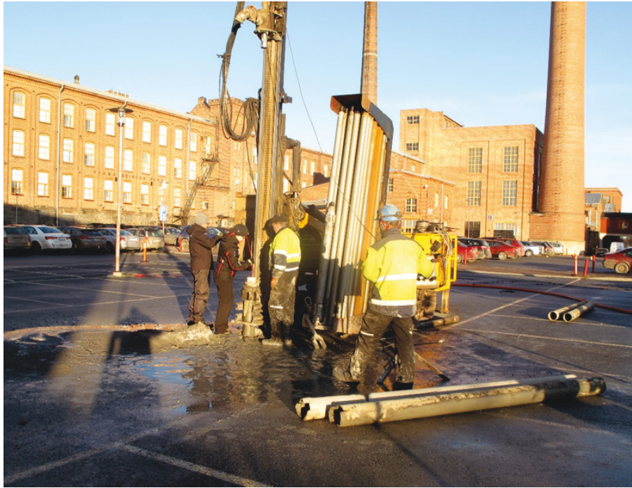
Figure 3. Drilling of measurement field at UVA campus area in November 2013.
