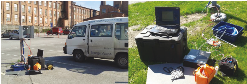
Figure 8. Splice box with connectors in the asphalt field and DTS device, laptop, calibration coil and battery.
