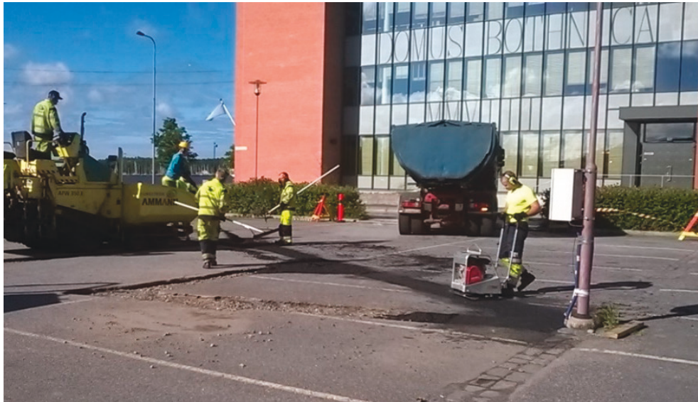
Figure 2. The measurement field receives asphalt pavement after drilling and digging.
