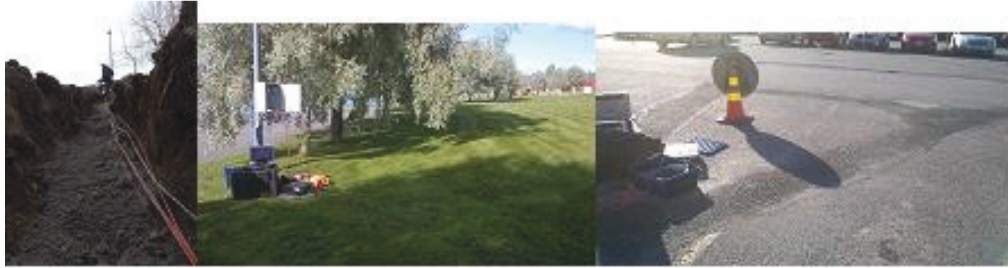
Figure 6. The implementation of cables and the completed measurement fields.
