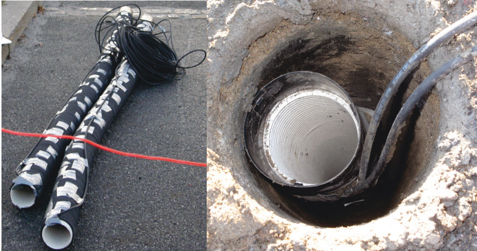
Figure 4. Cables were wired around drainpipes (diameter 100 mm) in the 3 m-deep holes.
