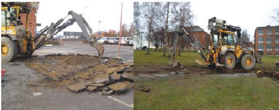
Figure 5. Excavator was necessary in establishing the measurement field.
