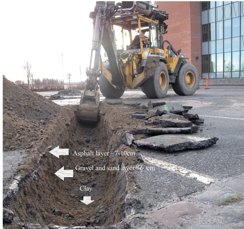
Figure 4: Soil layers under the asphalt in the measurement field.
