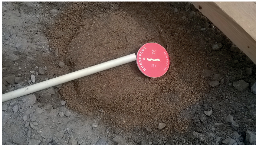
Figure 4. The sensor is placed just below the asphalt layer.
