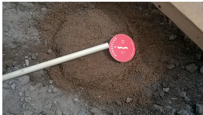
Figure 1: Installation of heat flux plate "Hukseflux".
